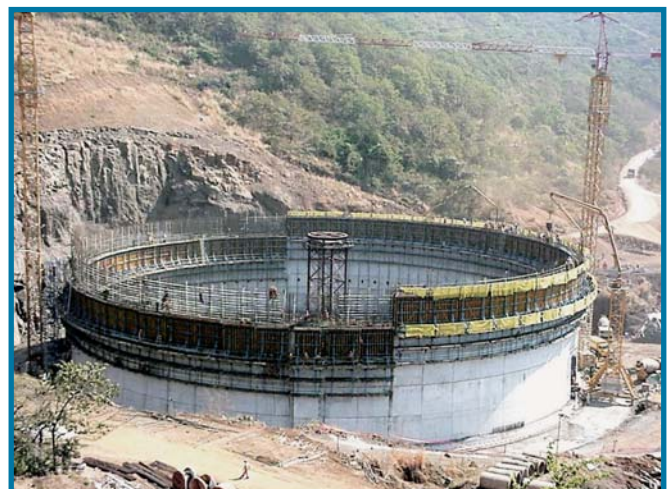
Fig. 1. Dabhol LNG terminal India, site overview of one of the three 9% Ni tanks that have been built by Skanska Whessoe according to the "double integrity concept" with a capacity of 163,000 \text{ m}^3 .
