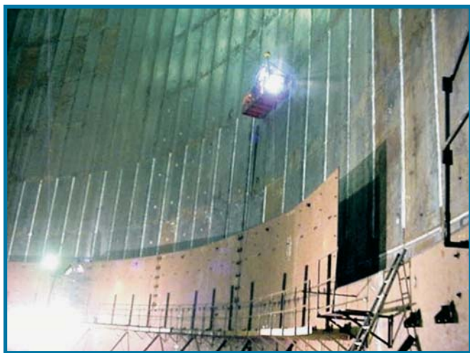
Fig. 2. Dabhol LNG terminal India, inside view of the construction of the 9% Ni steel inner shell and the concrete outer shell for one of the three tanks built by Skanska Whessoe according to the "double integrity concept" with a capacity of 163,000 m 3 .
